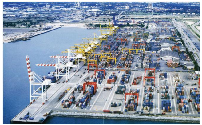
Figure 3 Laem Chabang Port construction – Phase 3.
